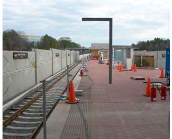
▼ Reston Town Center Station platform (train level) and looking easterly at the outbound tracks (out of DC). The concrete pavers are installed, the ADA strip, flashing lights along the platform edge, sign posts and wind screens.
