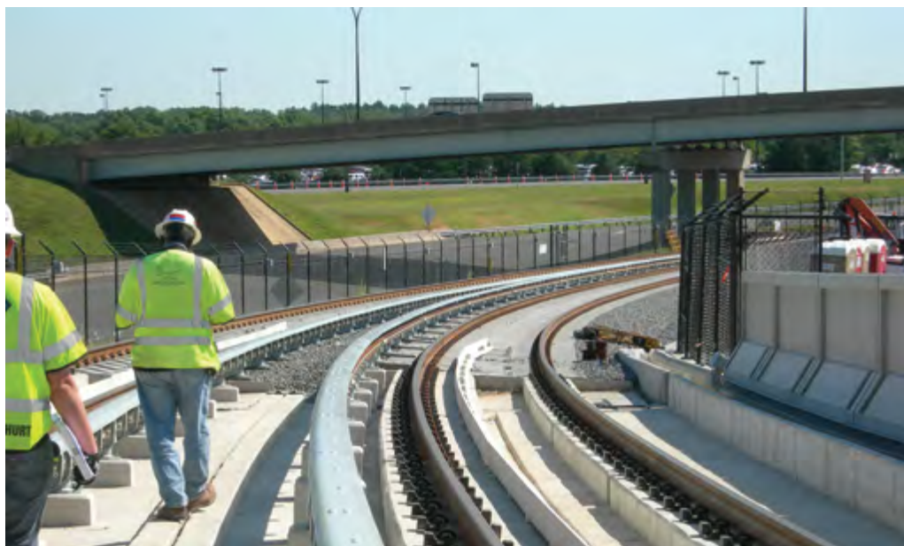
◀ Abutment A where the ballasted track (at grade) and the aerial guideway meet in the middle of the DIAAH on the Airport – looking to the south east. Rudder Road highway overpass goes over the ballasted track in the near distance.
