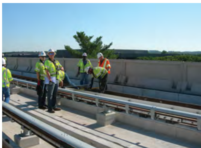
▲ The “Walk Down Team” reviewing the aerial guideway between Abutment A and the Airport Station. Checking the gauge of the tracks (distance between the rails), distance from the tracks to the third rail, visual alignment and overall condition. The sixth Walk Down with representatives from CRC, MWAA, WMATA and DRPT.
