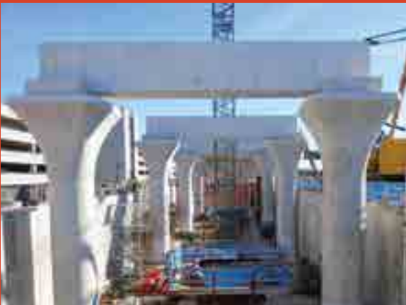
At Dulles Airport Station walls are being constructed. Station Columns and cross girders are being cast. Walk Back tunnel demolition has been completed and tunnel tie-in work started.
